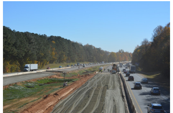
Aggregate rock placement in north segment
